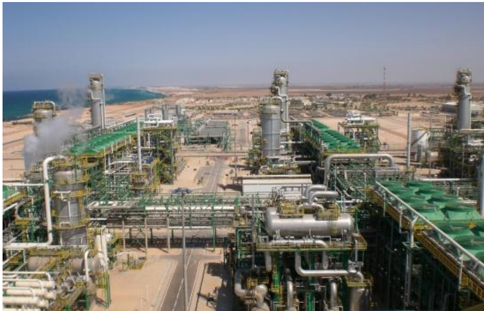
Mellitah Gas Plant Complex
